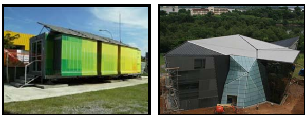
Figure 1: NAV mobile lab and LAMCE Construction.
