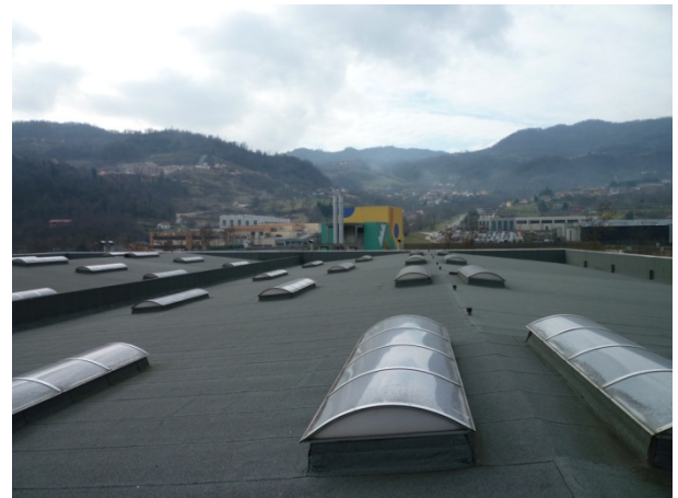
Figure 2: Top view of the T&T building double 5 deg gabled roof enclosed by a continuous brick fence
