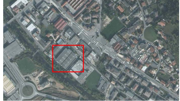
Figure 1: Aerial view of the T&T building site (the analyzed building is evidenced by the red rectangle)
