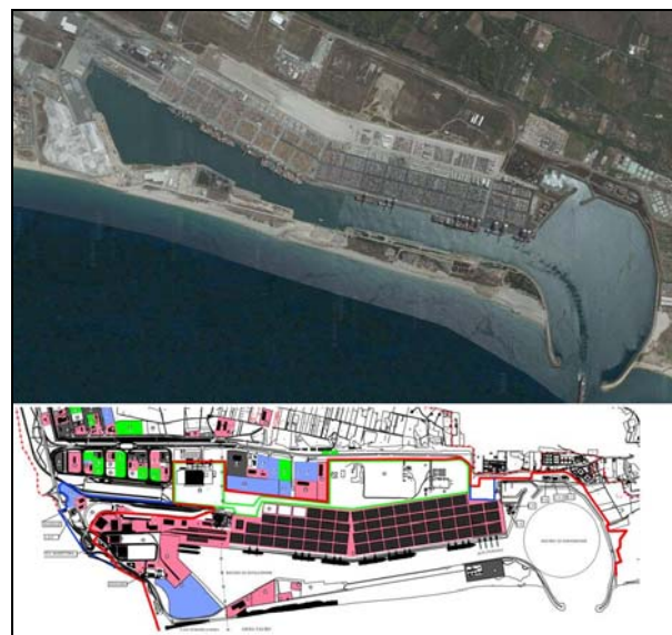
Figure 2: Panoramic view and lay-out of the Gioia Tauro Container Terminal
