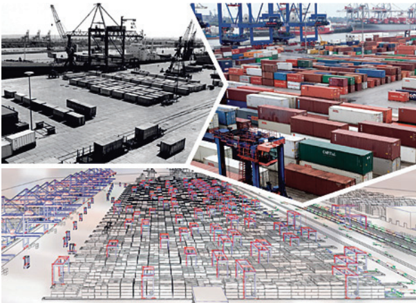
Figure 2: Progress in terminal operations: The Burchardkai, Hamburg, in 1968; straddle carrier based operation in 2005; and the future layout in 2014 with automated six-high storage blocks served by triple rail mounted gantry cranes (in red). Source: INFORM
