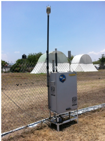
Figure 5. Air Pointer Monitoring Station Installed in the INAFAP
