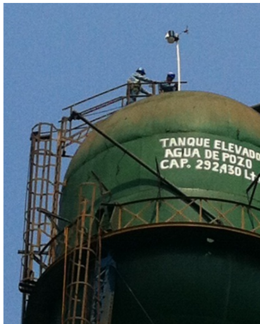
Figure 6. Installation of a DAVIS Meteorological Station in the Sugar Refinery
