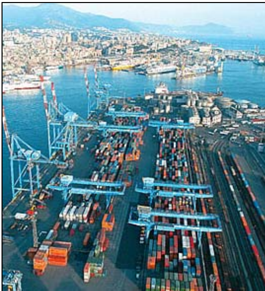
Figure 1: A view of Voltri Terminal Europe
