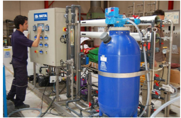
Figure 2: RO plant for testing.
