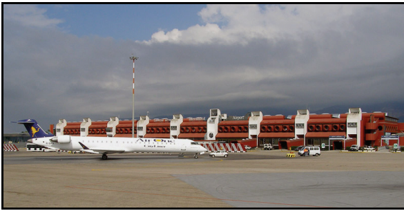
Figure 1: The Airport Terminal of Lamezia Terme
