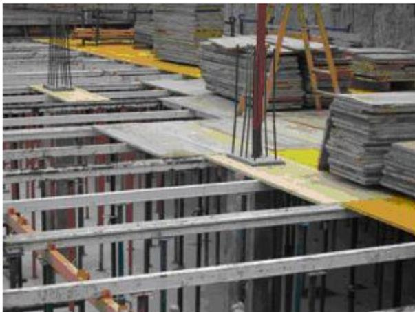
Figure 1 Provisional floorboard framework.
