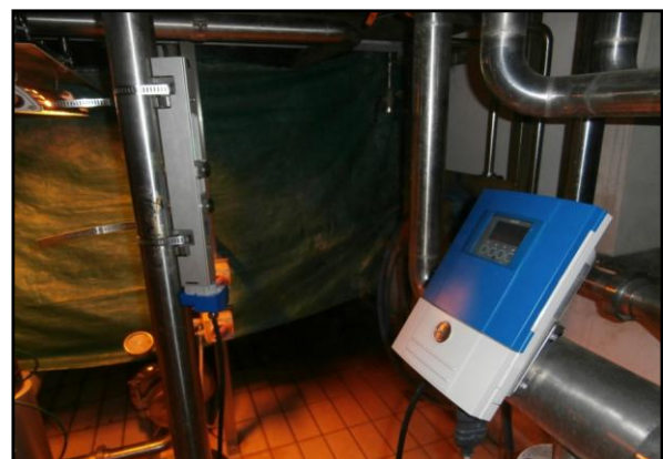
Figure 4 - Ultrasonic clamp-on flow meter
