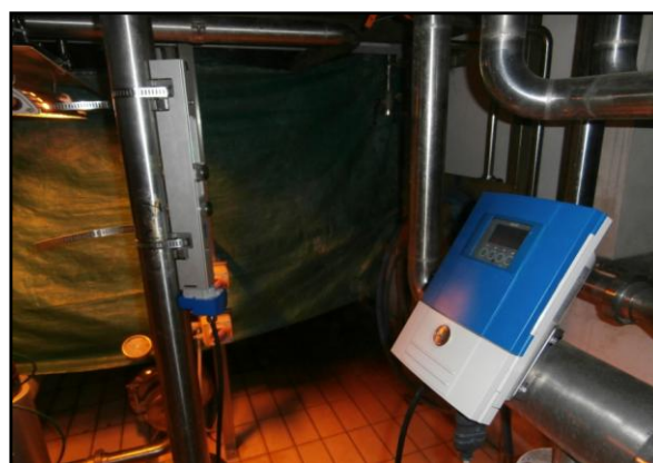
Figure 4 - Ultrasonic clamp-on flow meter
