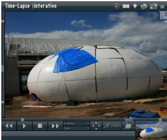
Figure 11: Timelapse Player screen showing the defective plates during the NVC assemblage.
