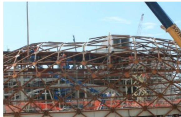
Figure 10: Close image of the NVC metal structure falling.
